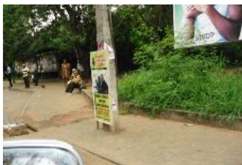
Figure 4: Sidewalk inhibited with potholes and poles
